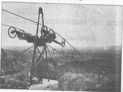
SINGLE ROPE TRAMWAY-Improved Type-Long Spans.
