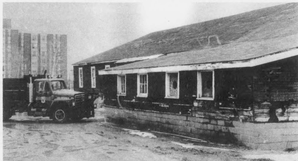
The Muskeg Building, currently used for maintenance storage, will be demolished to make way for the new daycare. Photo by P. DuChemin
