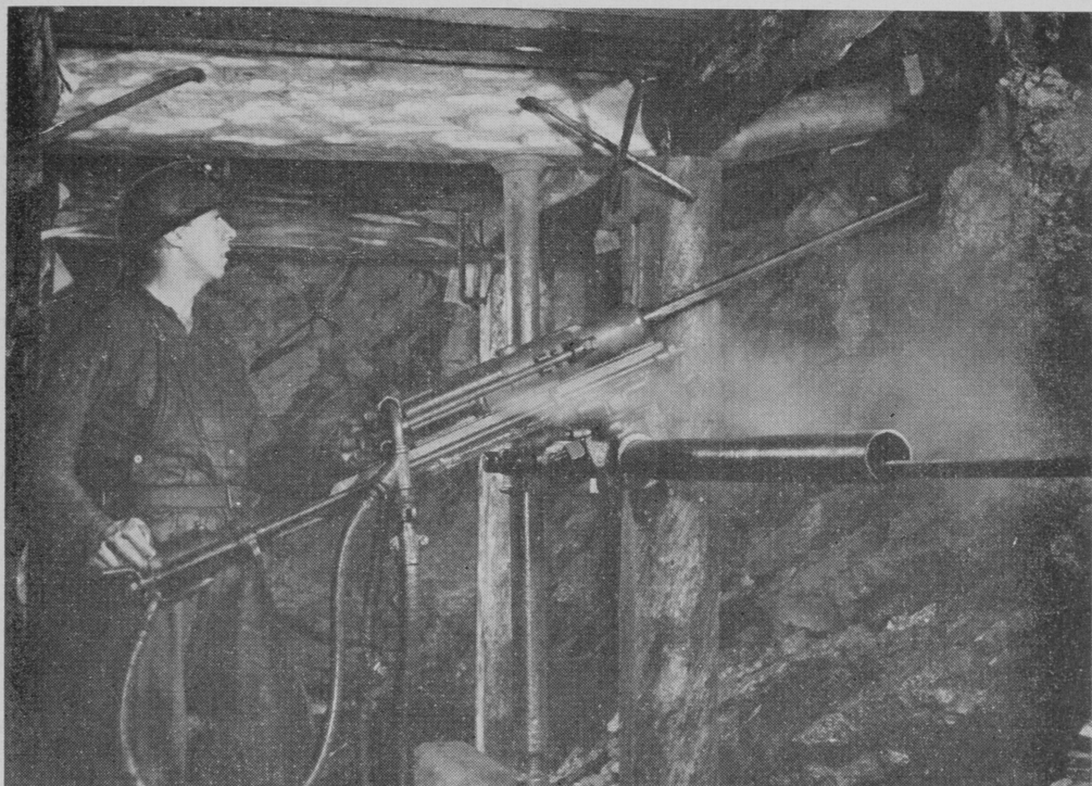
Drilling in square-set stope, Frood-Stobie Mine.
