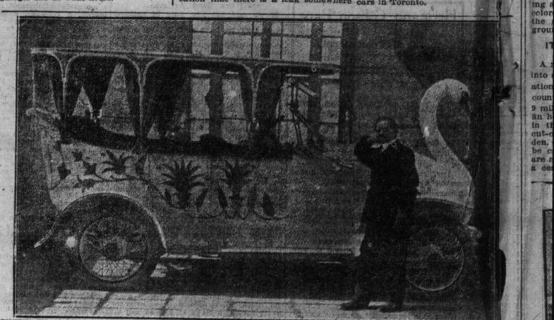
SUITED TO A UP-TO-DATE LOHENGRIIN, A SWAN-SHAPED MOTOR CAR, WHICH, AS DOES THE BIRNIT RESEMBLES. This remarkable car, made for use in India, cost \$12,000. It has electric-light eyes. The exhaust can be sent thru the beak, causing the "swan" to hiss.
