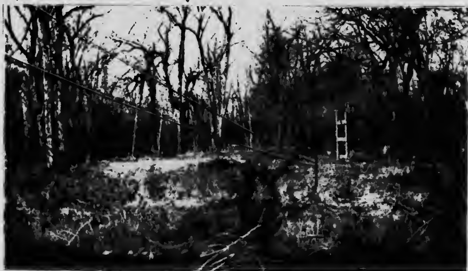
Ochre River at Ochre River—Meter Section. Showing installation of Cable Carrier.
