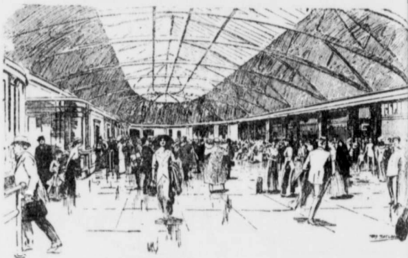
Concourse, Windsor Street Station, Montreal
