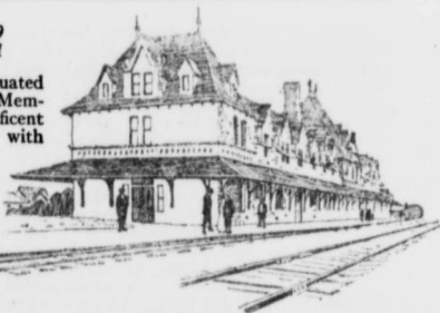
Station and Hotel, M. Adam Jct., N.B.
