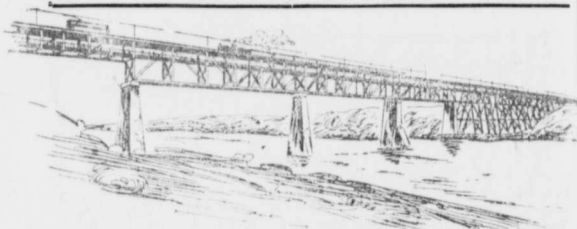
C. P. R. Bridge over the Saskatchewan River at Edmonton
