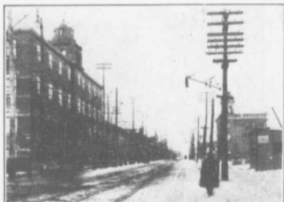
VIEW OF ONTARIO STREET
