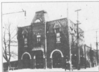
No. 1 POLICE &amp; FIRE STATION.
