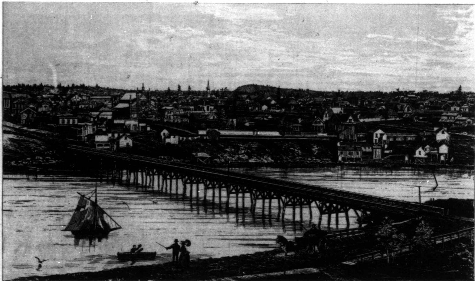
JAMES BAY BRIDGE, VICTORIA, B. C.
