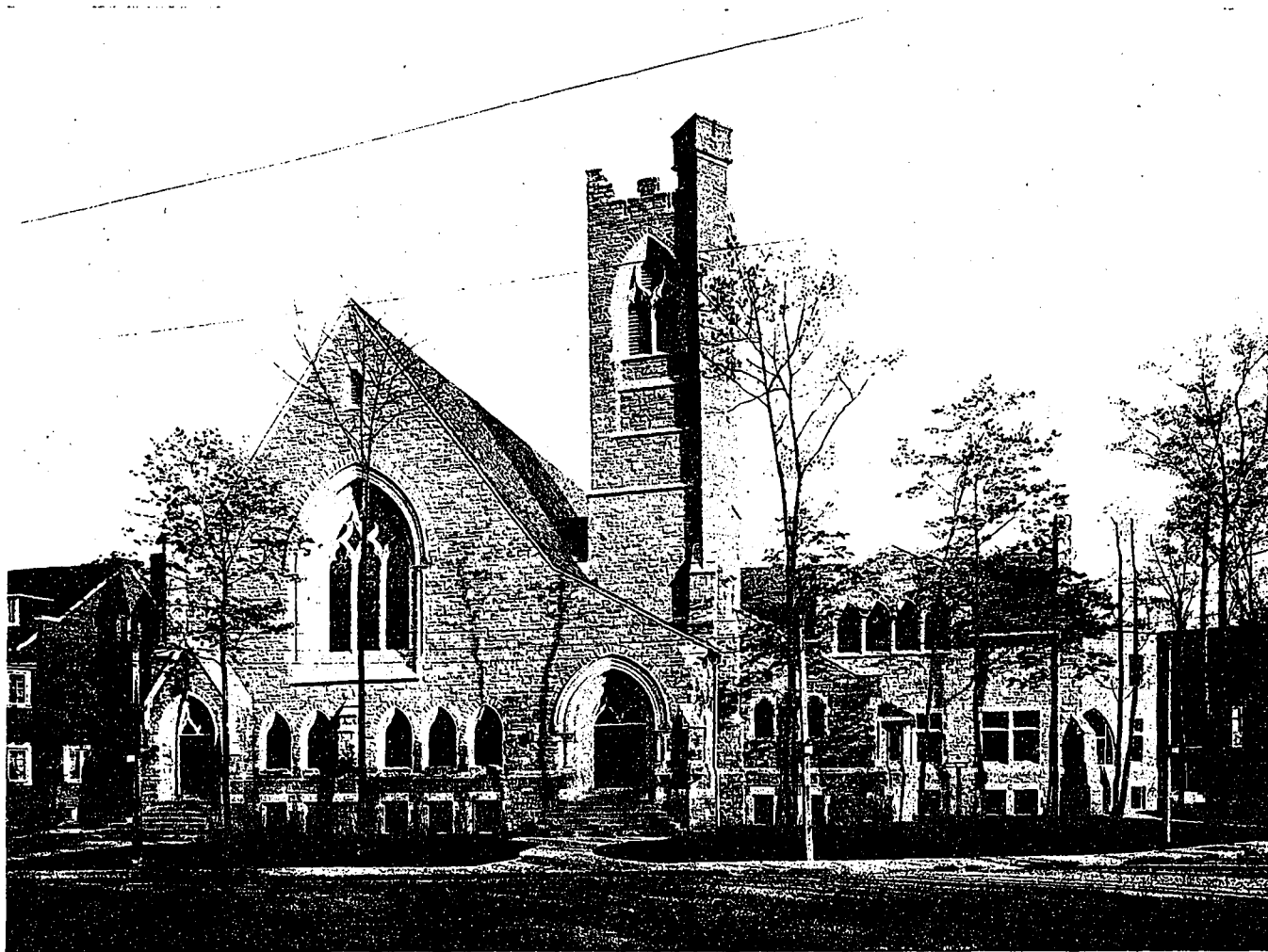
NORTHERN CONGREGATIONAL CHURCH, TORONTO, ONT.
