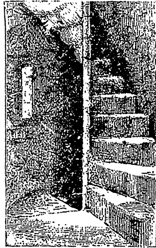
STAIRWAY, HOLYROOD PALACE.
