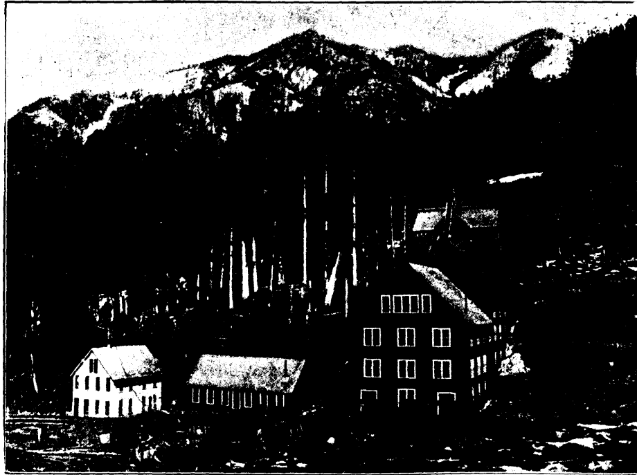
THE CONCENTRATOR AND TRAMWAY—NOBLE FIVE MINE.
