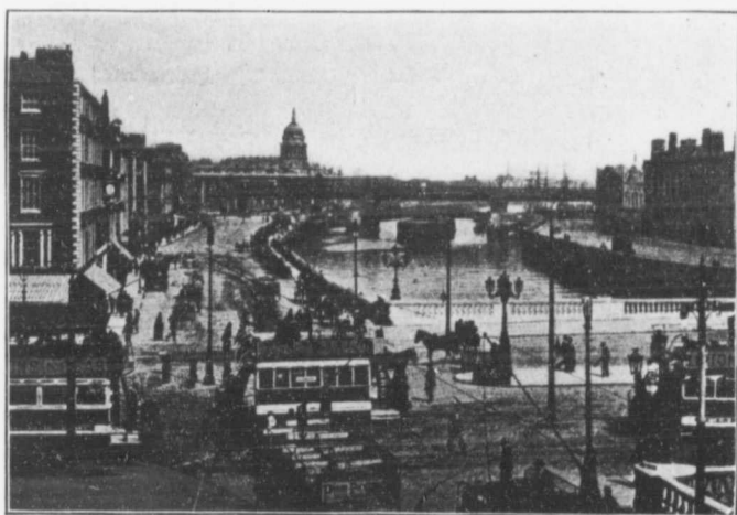
O'Connell Bridge, Dublin.
