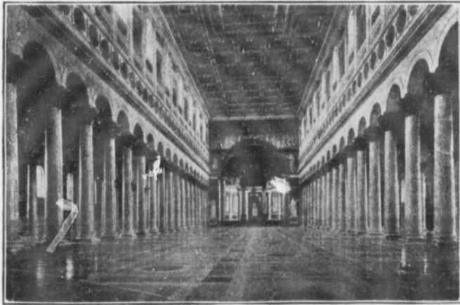
Interior of St. Paul's, Rome.
