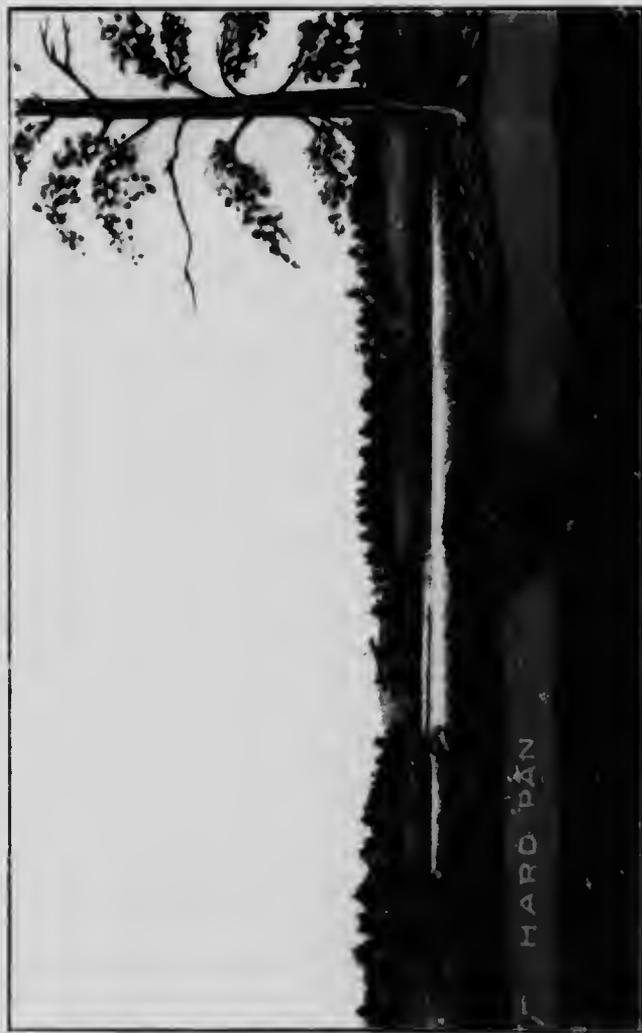
Section Through Haropan, Showing Effect of a Quick-Acting Explosive
