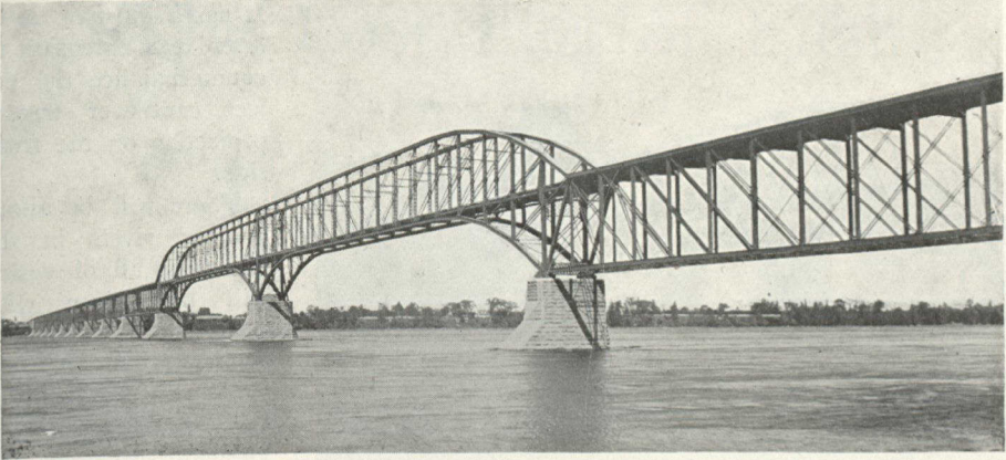
C.P.R. BRIDGE OVER ST. LAWRENCE RIVER AT MONTREAL Commenced 1887. Weight 8,200,000 lbs. Single track. Opening below cantilever spans, 60 feet.
