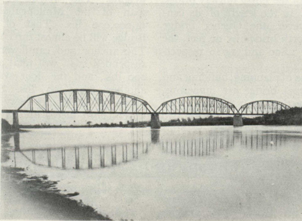
THE SOUTH BRIDGE AT CORNWALL ISLAND
