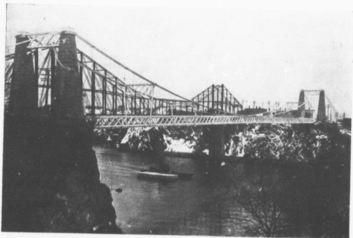
REVERSIBLE FALLS, ST. JOHN, HIGH WATER. The falls are navigable during high water. The bridges are the Suspension and C.P.R. Cantilever.
