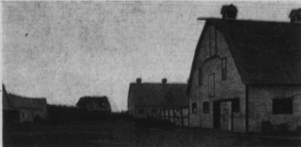
Farm Buildings and Home of Capt. A. R. Gillies, Clover Bar, Alta. These buildings are all equipped with Electric Light, and all other Modern Conveniences and Labor-Saving Devices.
