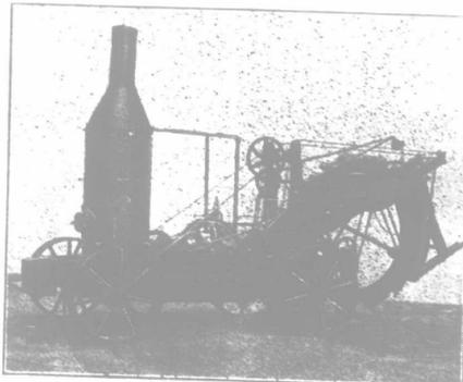
Every farmer and thresher-man knows the value of a time-saving machine such as a harnessing machine. We want YOU to know the money making qualities of the BUCKEYE TRACTION DITCHER. It cuts 100 to 180 feet per day, and saves 25 per cent to 50 per cent of the cost of handwork. Are YOU interested? Write TODAY for catalogue. Remember the first man in your vicinity to use a BUCKEYE will make the biggest profit. Address:
