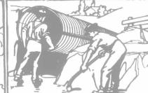
These pictures show how easily and quickly you can lay Pedlar Culvert. Comes nested, half-section within half-section...-saving freight and cartage. Triple-thick Flat flange locking ribs on each side are clamped together by a simple tool---no bolts nor rivets needed. Joints are broken.—only culvert you can do that with. Ends interlap. Will stand tremendous strains. Won't leak, nor buckle, nor crack from frost. Cheaper than wooden culverts
