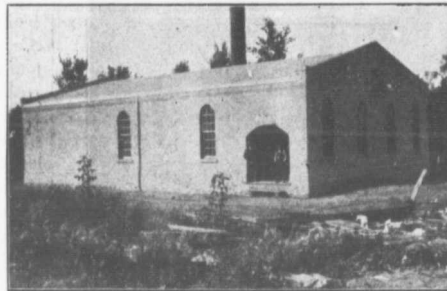
ELECTRIC POWER STATION, DAUPHIN, MAN.
