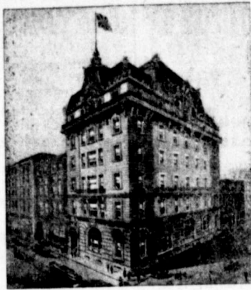
COMPAN'S BUILDING, MONTREAL.
