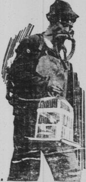
of the rescuers with oxygen equipment and a canary. Poisonous gas quickly kills the bird. Miners without helmets are not permitted to enter chambers where the canary cannot live.
