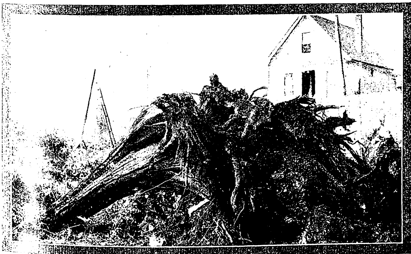
AFTER THE CHARGE HAS SPLIT THE SOLID STUMP FROM BASE TO SUMMIT
