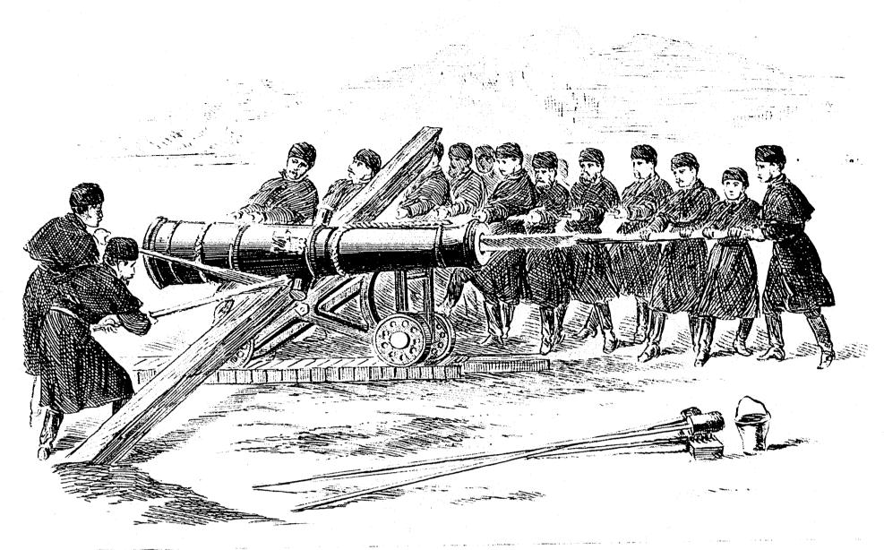
MOUNTING A 52 CWT, 32-POUNDER, ON AN IRON CARRIAGE BY A SINGLE TIMBER UNDER THE CENTRE OF GRAVITY
