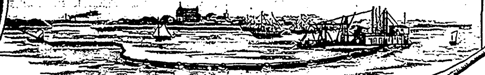
HYDRAULIC DREDGE DISCHARGING THROUGH ONE HALF MILE OF PIPE.
