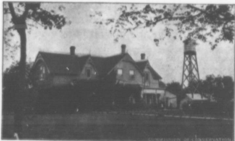
In this house there is water on tap. The windmill on the barn is geared to elevate water to the raised tank. Note that the well is protected by the pump house.
