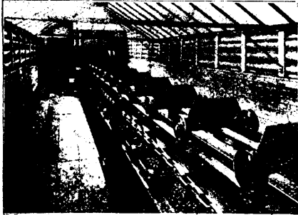
Coal and Ashes Handling Machinery
