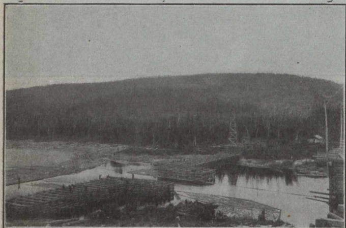
Upper West Cofferdam Under Construction, Looking East
