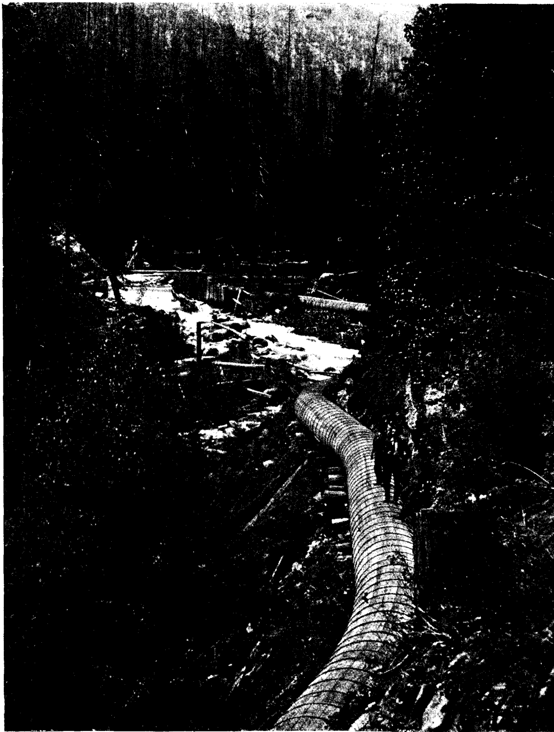
Pipe-Line Taylor Air Compressor Plant at Ainsworth.
