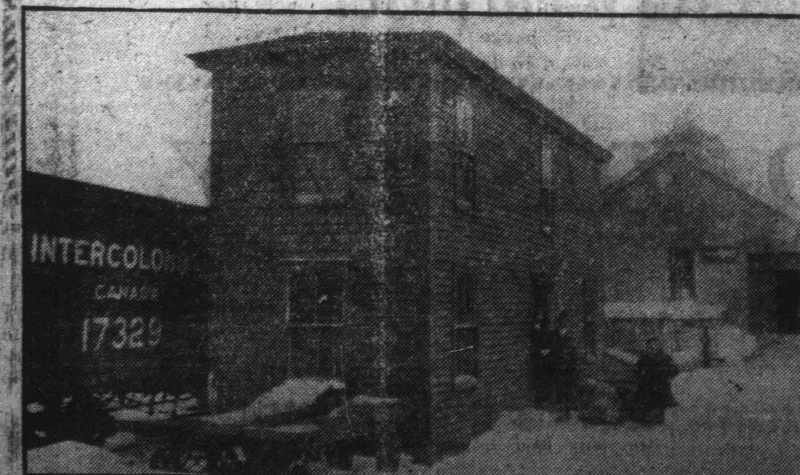
Newfoundland Government Post Office Shack at North Sydney.
