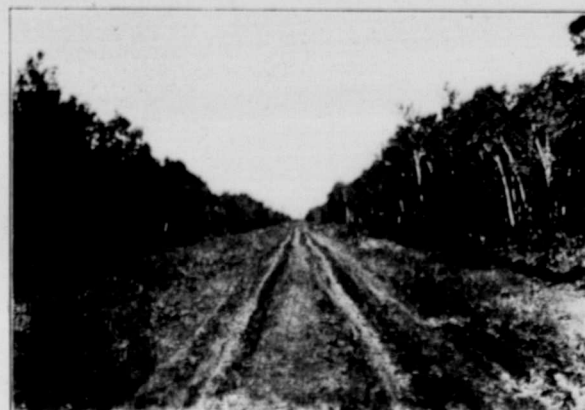
Split-log drag kept this road well rainproof but was neglected after a rain and was soon in poor condition. Drag would have removed ruts.
