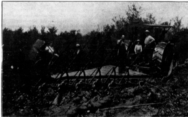
Plowing with a "Stover Tractor" on the Farm of Ivan Dacock, near Deleau, Man. A Big Dutchman Engine Gang made by the Moline Plow Company is turning the furrows.
