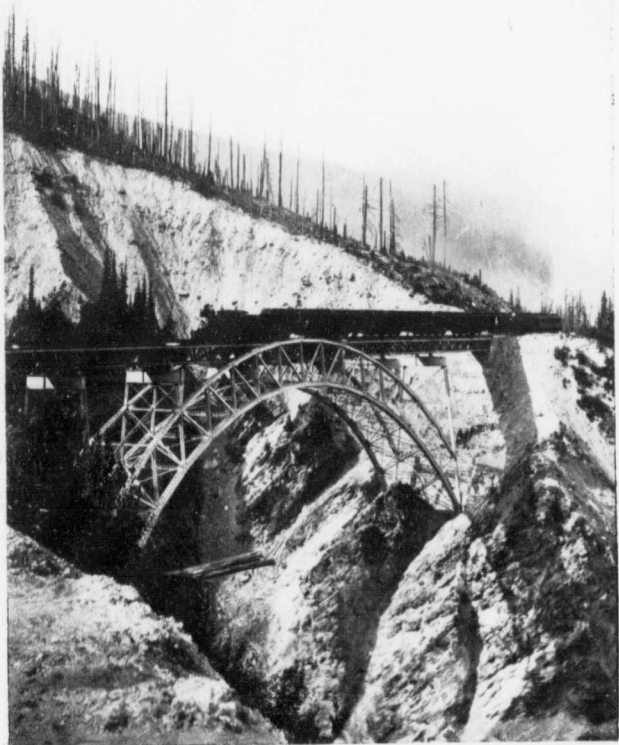
STONY CREEK BRIDGE, BRITISH COLUMBIA.
