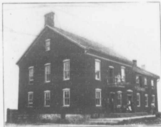
The Ontario House.
