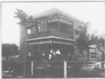
Residence of Chas. Wilken.
