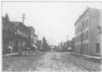
View of Arthur St.,—southward.
