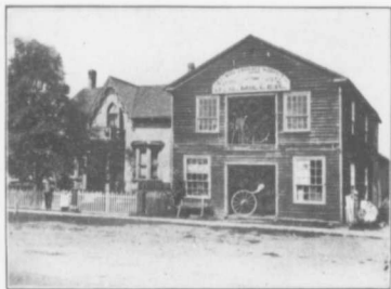
Residence and Carriage Shop of J. S. Miller.
