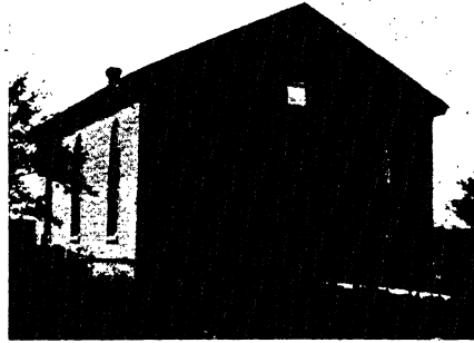
Methodist Church, Port Robinson
