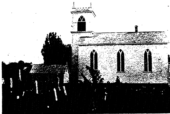
St. Paul's Church, Port Robinson
