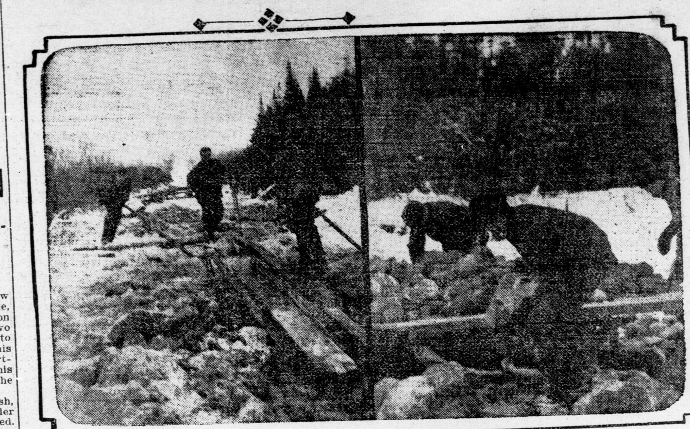
(By Staff Photographer.) 1. Getting out sleigh, which has sunk from sight, all but pole. 2. Unloading "hard heads" in effort to make foundation for filling.
