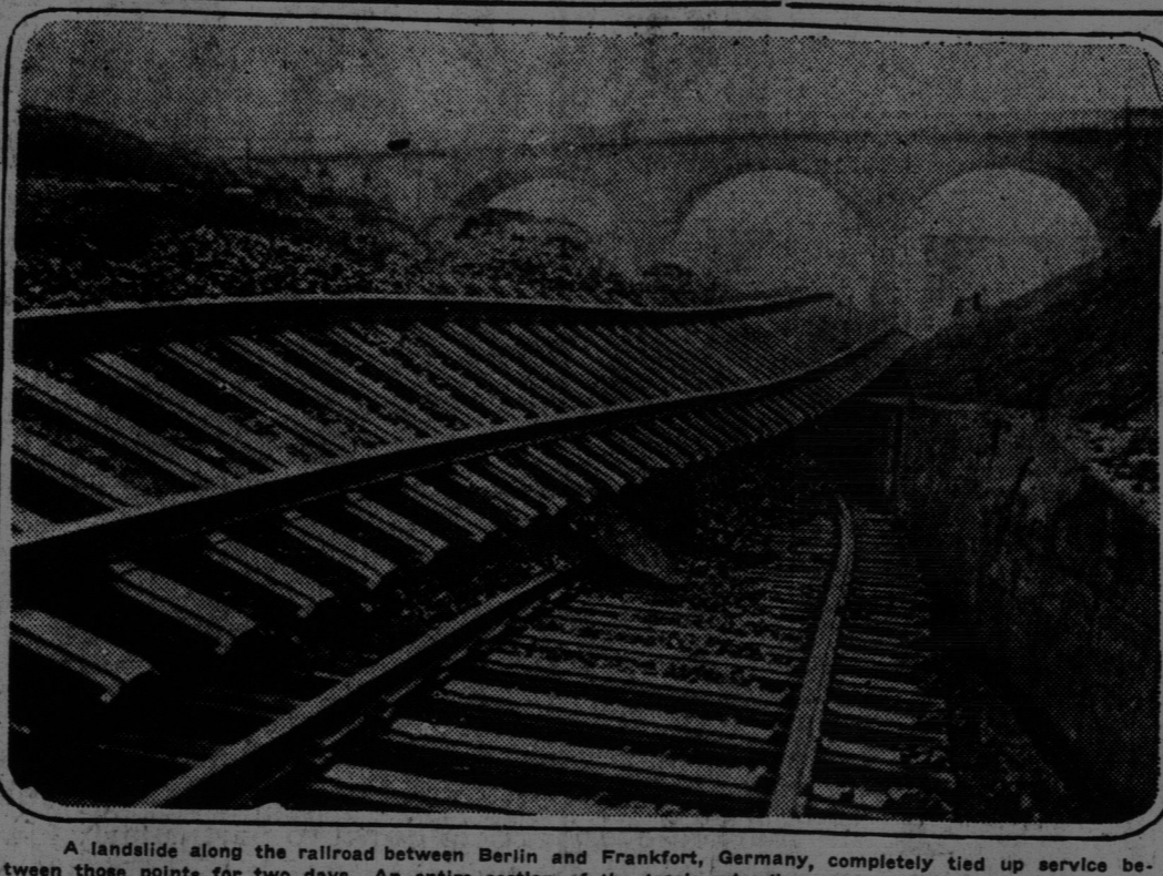
A landslide along the railroad between Berlin and Frankfurt, Germany, completely tied up service between those points for two days. An entire section of the track extending nearly a quarter of a mile slid down to another section of the rails, tying up traffic in both directions. Above is a view of the landslide.
