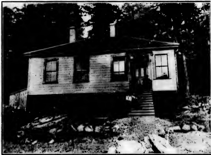
Government Building at Jedway. Municipal Offices.
