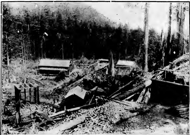
Entrance to Tunnel No. 1, Ikeda Mine, Ikeda Bay.
