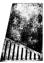
FERRO-DOVETAIL PLATE CONCRETED ON TOP, PLASTERED UNDERNEATH
