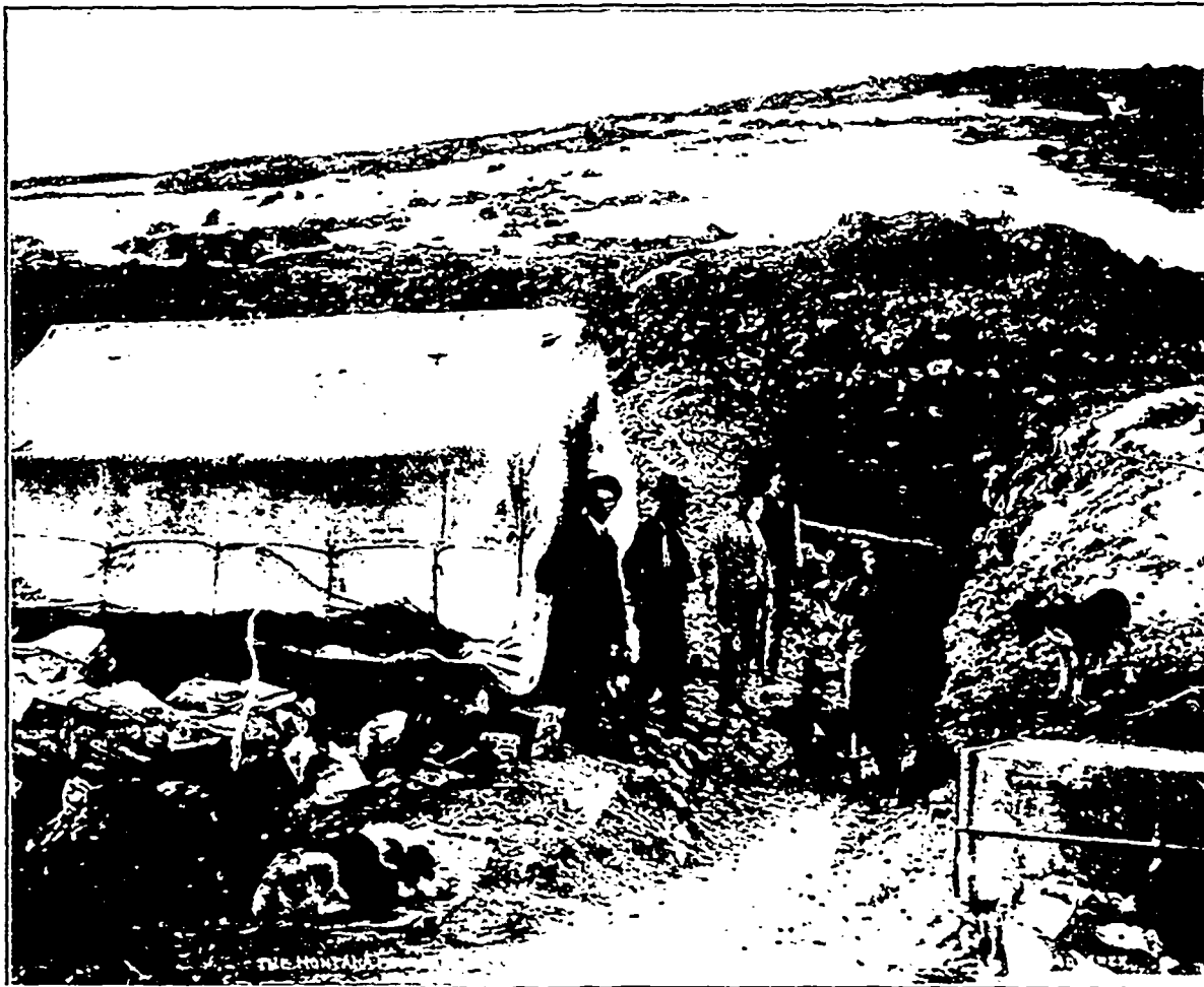
Entrance to Tunnel on Montana Claim.—Length of Tunnel in October, 360 ft.
