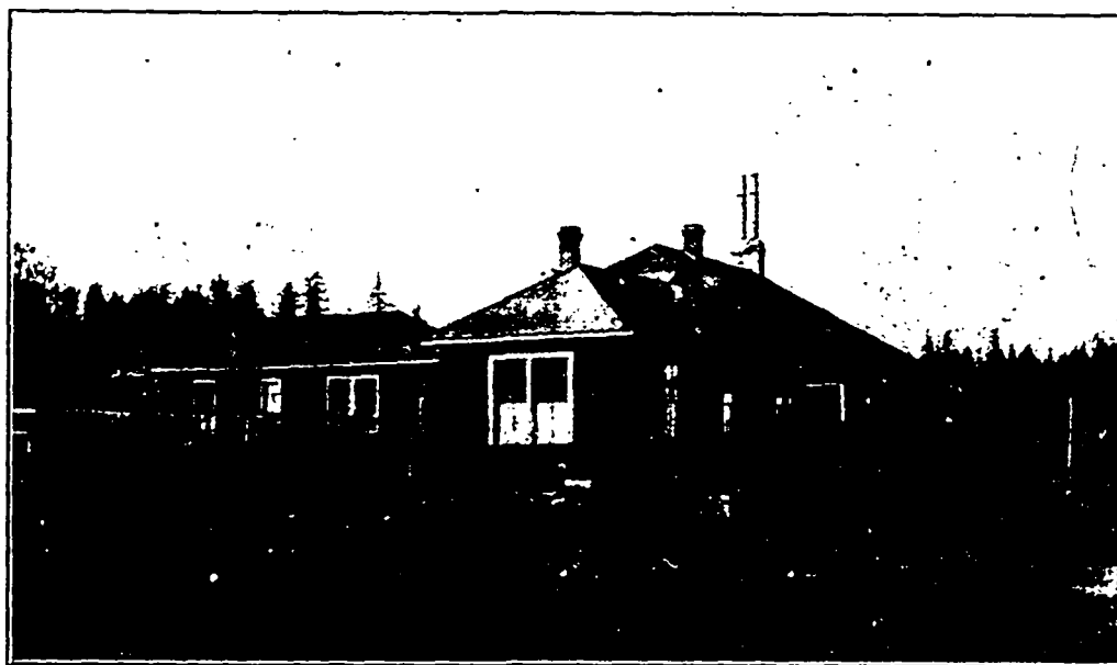
Britannia Smelting Co's Smelter.—General Offices at Crofton.
