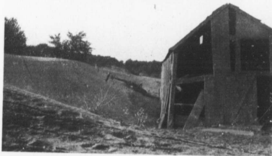
AN ABANDONED FARM SHOWING EFFECTS OF DRIFTING SAND.
