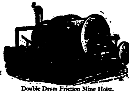
Double Drum Friction Mine Hoist.
