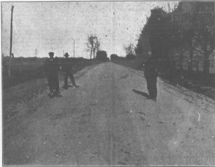
A BROKEN STONE ROAD BUILT LAST YEAR
