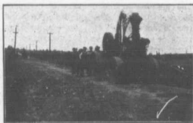
Consolidating the Metal
