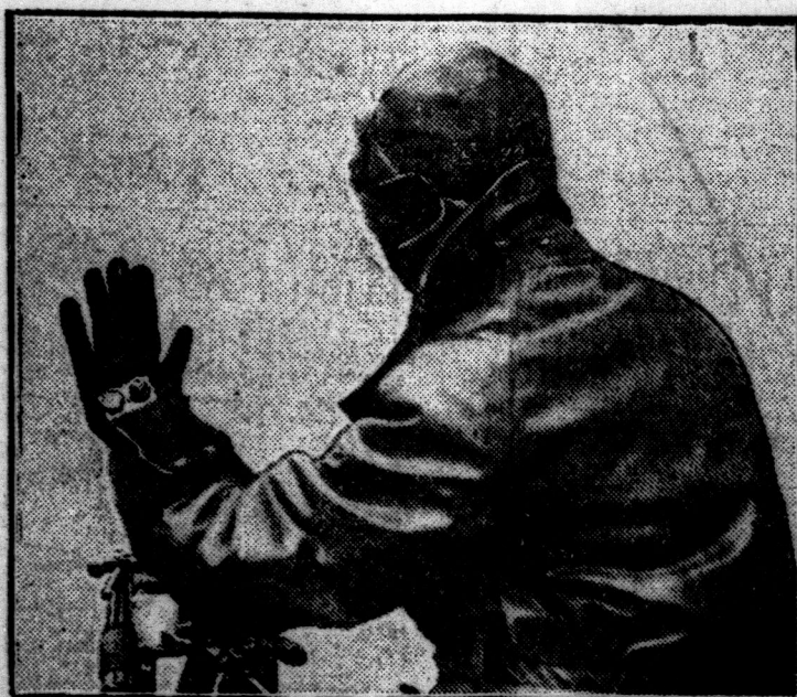
An illuminated glove was one of the many novelties seen at the cycle and motor cycle show, Olympia, England. The glove is fitted with a red and white lamp for signal purposes
