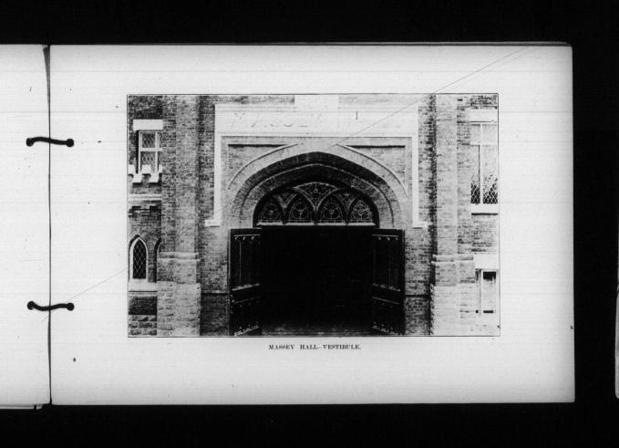
The basement walls are built of logal limestone and all exposed portions carried out in coursed rock-faced masonry. The superstructure is of red brick, liberally trimmed with Ohio freestone, finely chiselled.
