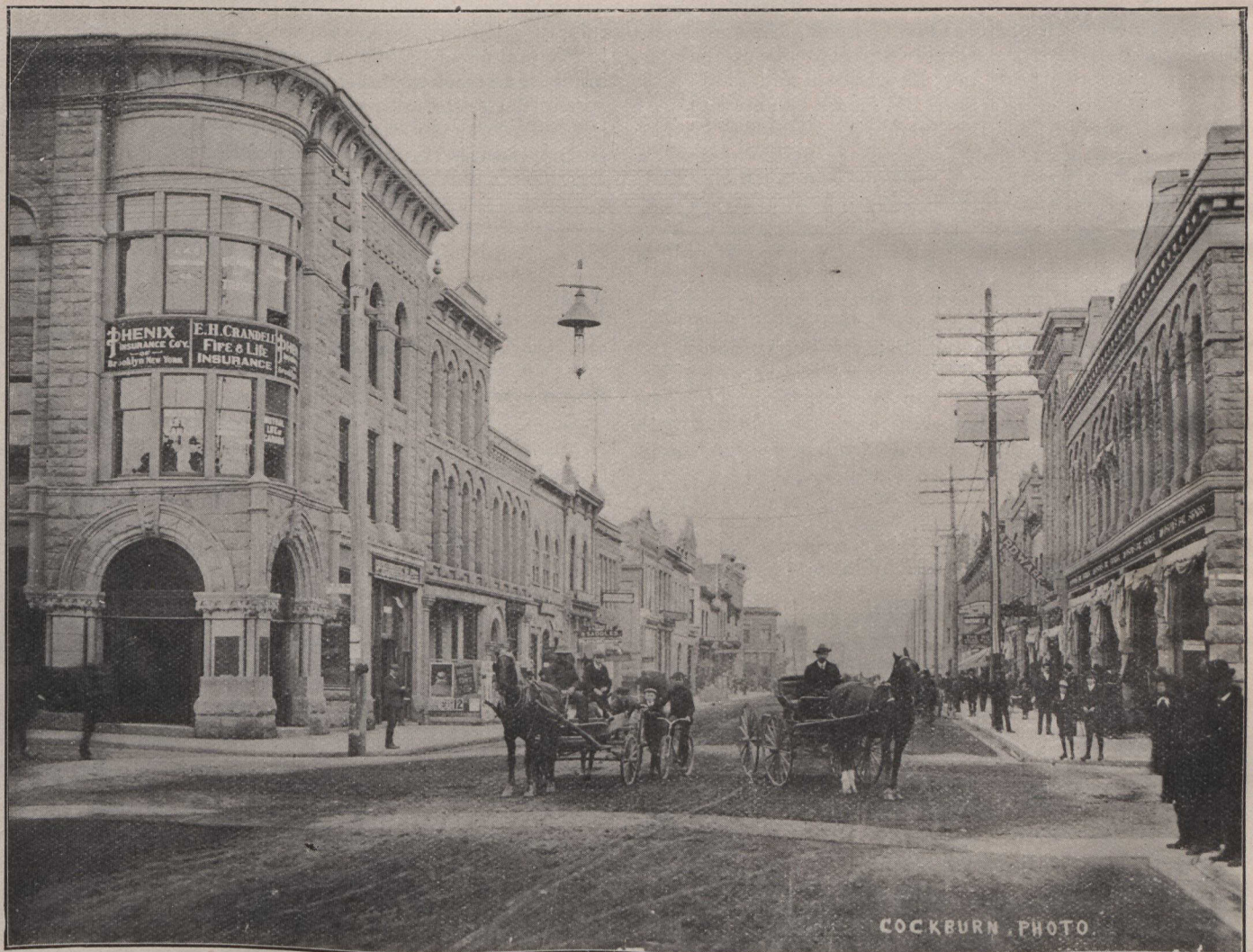
VIEW OF A PORTION OF THE RETAIL SECTION AT CALGARY
