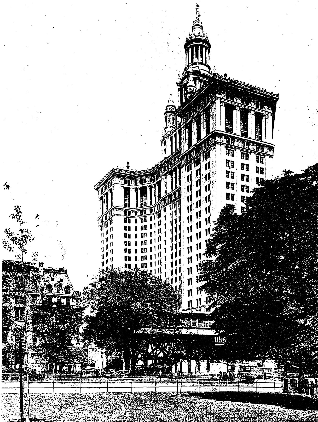
MUNICIPAL BUILDING, NEW YORK CITY.
