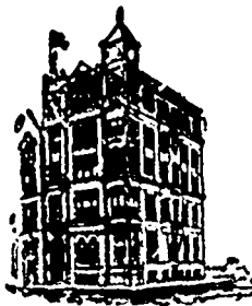
HEAD OFFICE BUILDING, MONTREAL.
