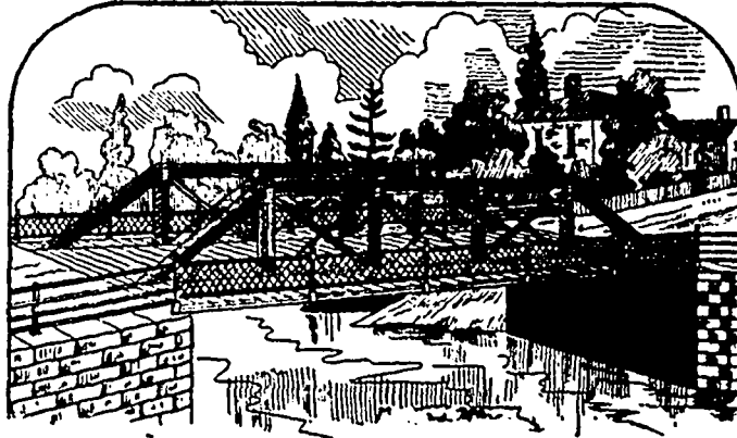
THE NEW PIGEON CREEK BRIDGE.
