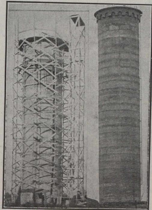
those in foundation, and  $\frac{5}{8}$ -in. horizontal rods spaced according to pressure requirements, from 8 rings at the bottom to 3 rings at the top for each foot of height. About 35,000 lb. of steel was used for reinforcement.
