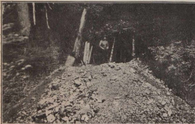
Lulu Tunnel—Glacier Creek Mining Co.
